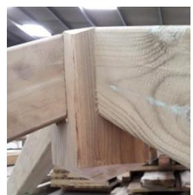
Predrill and with the 100mm screws, affix the eight corner braces (part 7), one end against the leg and one end against the top beam.
