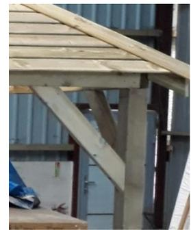
Roof boards (parts 10). Start with the four longest ones (2775mm) and fit them at the bottom of the purlins overhanging by about 20mm, leaving 3 to 4mm gap where the boards meet each other. Once this is done correctly, the rest of the boards should fit nicely all the way up to the top. Affix these with the 8 x 1/12 screws
